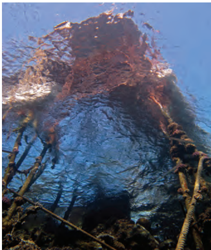
Wide angle image of a jetty structure.
